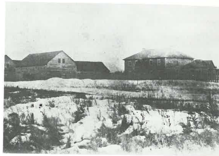
FIG. 38—Fort Ellice in its later years. Note the Red River cart near the building on the left.
