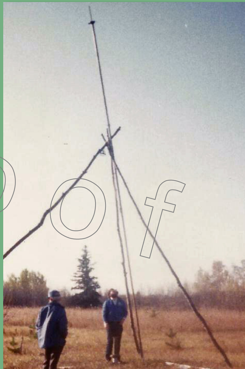
Helping Marvin pull the handpump from the well
